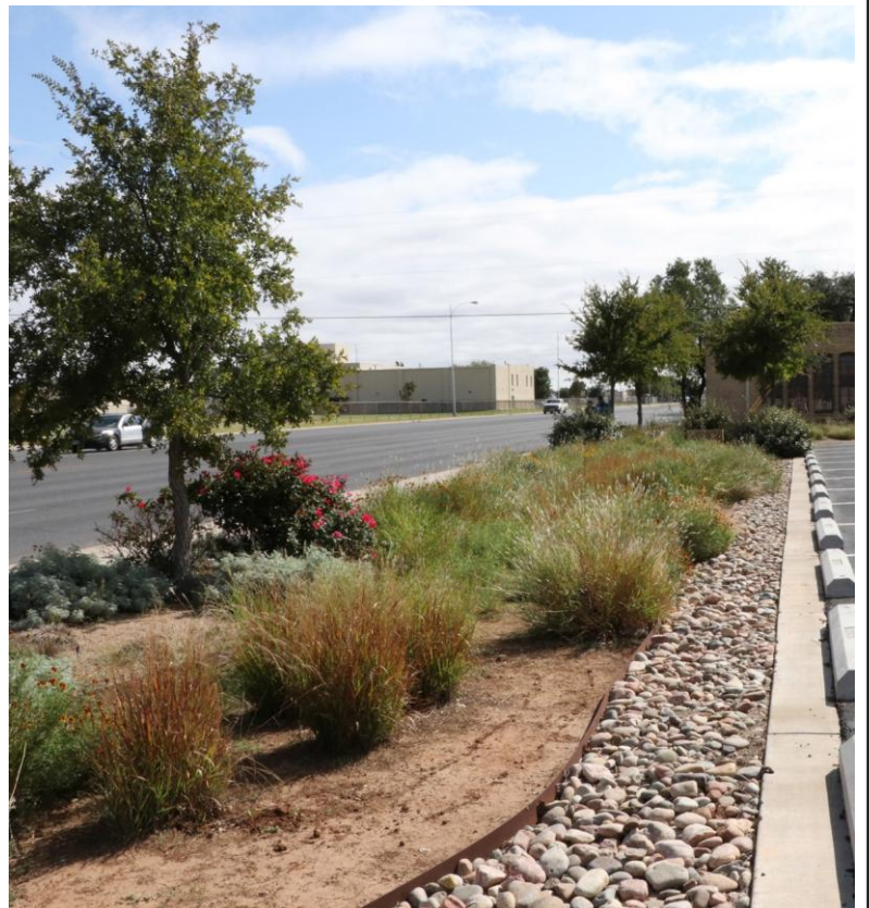
The rain garden at the High Plains Underground Water Conservation District Office (29th Street and Avenue Q) can catch 5,000 gallons of rainwater.
