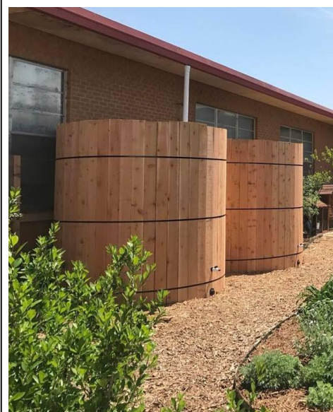
Two 2,500-gallon black poly tanks at South Plains College in Levelland were wrapped in cedar planks to make them more aesthetically pleasing.
